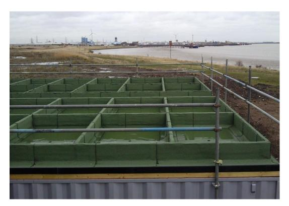
Figure 3. Completed green roof test bays with water proofing at Barking Riverside Offices.
